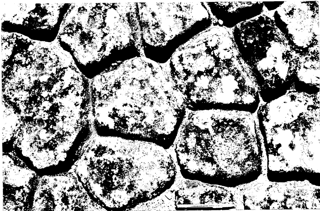
Figure 14: Polygonal thermal cracks in the upper surface of the sandstone plateau with profusion of lichens aiding disintegration and erosion.
