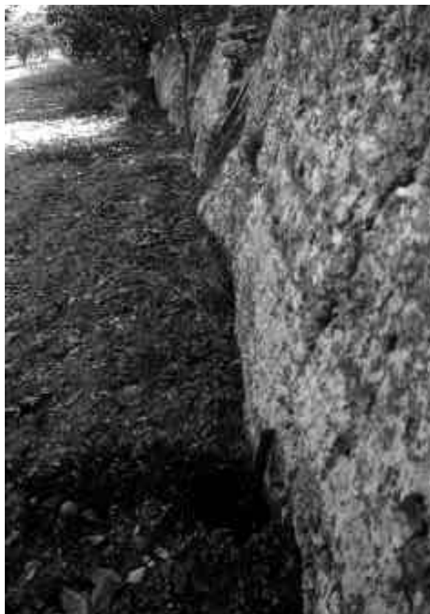
Figure 7. Detail of the two basal differentially weathered fault ribbons in the western sector of the Sta. Eugènia bedrock fault scarp (Sencelles fault). Hammer for scale is 33 cm long. Note that the hammer is within an artificial exploration scour 15 cm depth.
