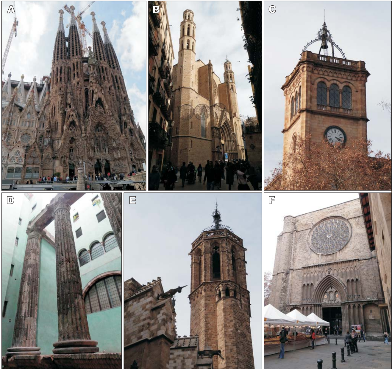
FIGURE 3. Examples of monumental buildings in Barcelona built with Montjuïc stone. A) Sagrada Família Temple (XIXth century). B) Church of Santa Maria del Mar (XIVth century). C) Historic building of the Universitat de Barcelona (late nineteenth century). D) Roman Temple of Augustus (first century B.C.). E) Barcelona Cathedral (XIIIth to XVth centuries). F) Church of Santa Maria del Pi (XIVth century).
