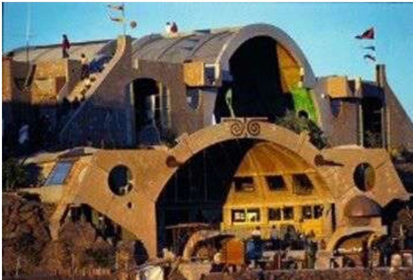
[Fig. 38] Apse workshops at Arcosanti. Courtesy of Pinterest.
