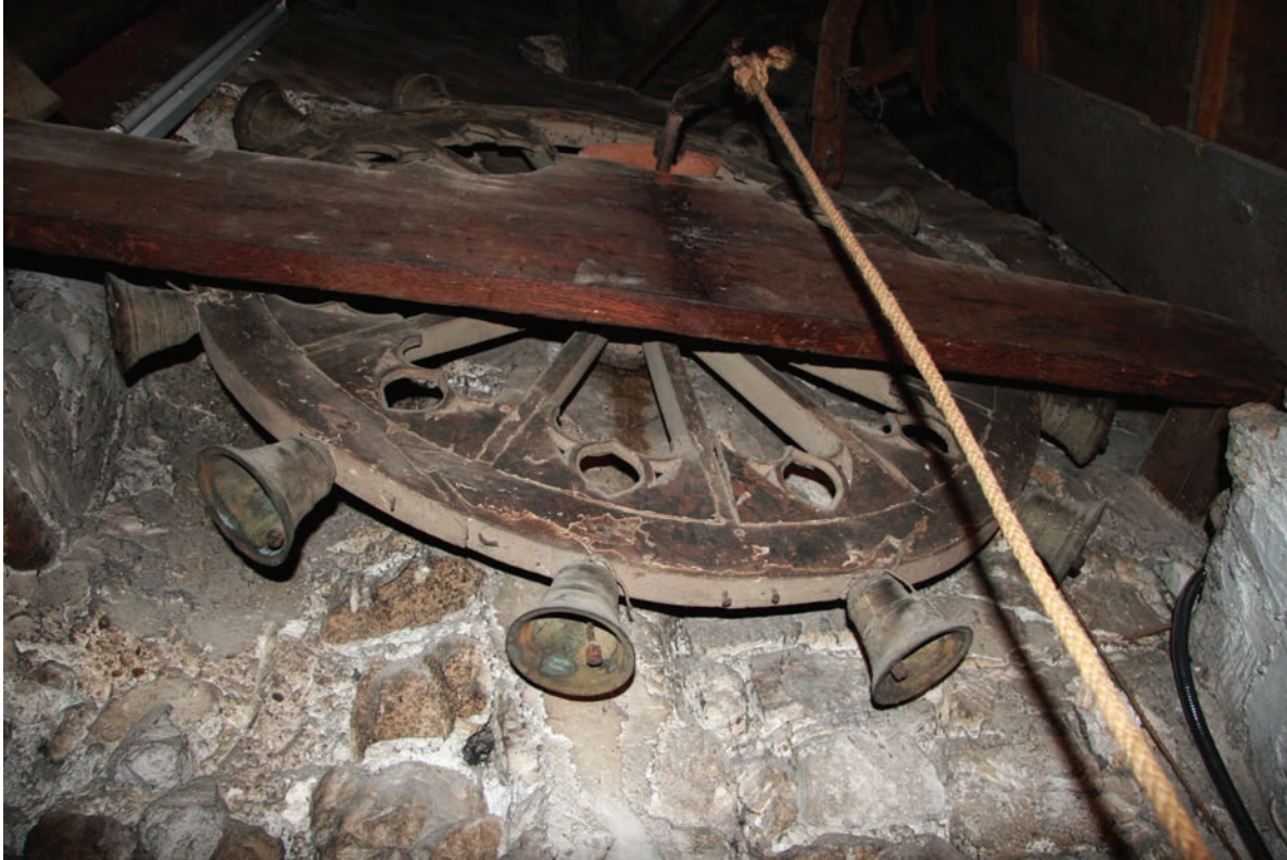
Fig. 11 Bell wheel, church of Our Lady of Angels (Pollença). Only the central piece of the bell wheel has been preserved and the wheel spokes feature and openwork pattern outlining pointed arched windows. Photo: Online digital archive ( www.campaners.com [2018/04/20]). Association of Bell Ringers of Valencia. Author: Pep Aspas Peris.
