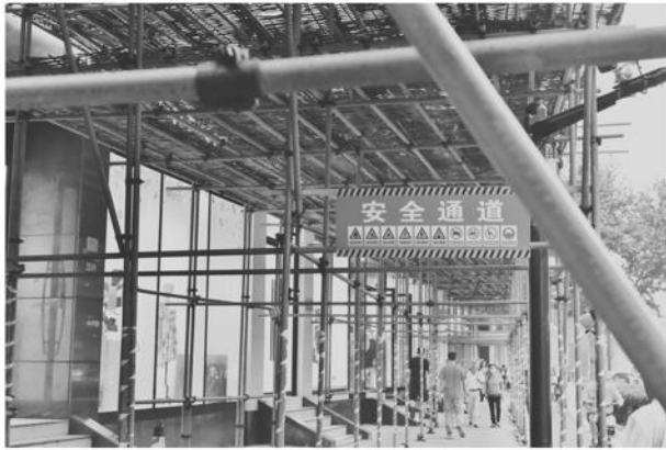
Figure 1. a construction site
