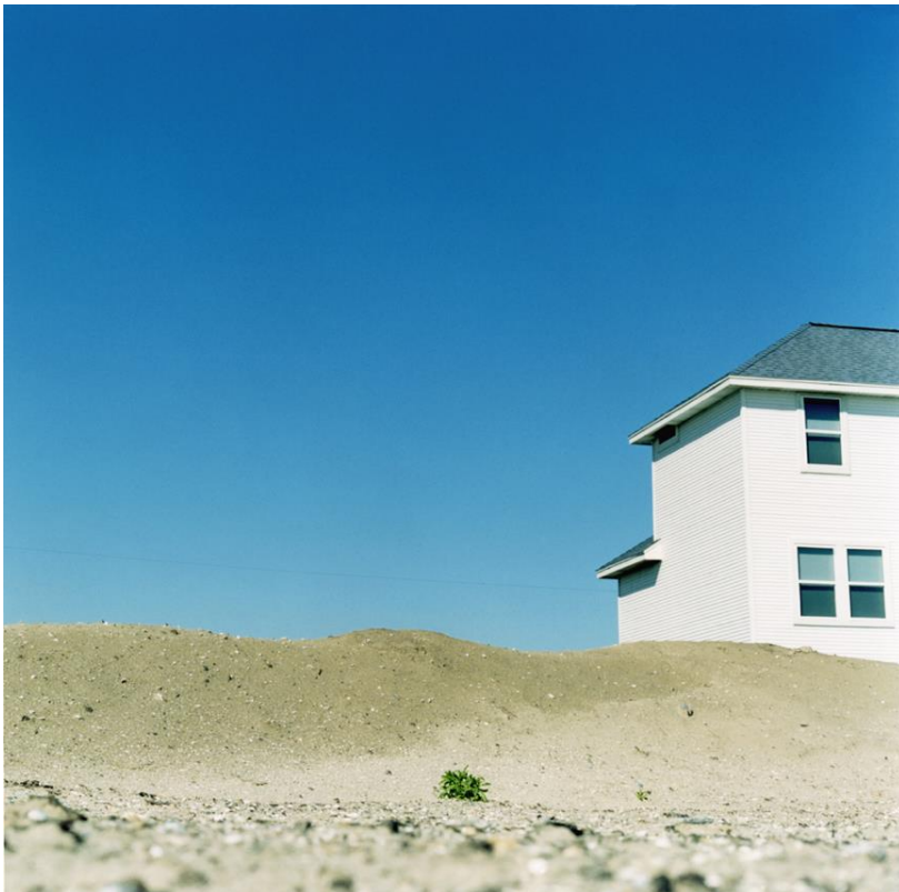
Land Development Site #03, Galveston, Texas, USA. Photographic Chromogenic Print of housing construction site on the island of Galveston, Texas (Edition of 50). 7.5x7.5 inches
