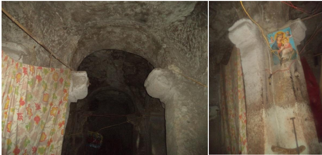
Figure 8 (left). Partial view of arched pillars. Source: author (2015).
