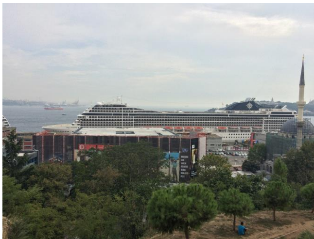
Figure 6. View towards the port: The cruise antrepo together as a symbol of socio-cultural transformation in the historical landscape. On the left is Antrepo no. 5 by Sedat Hakkı Eldem, transformed to Sanat Limanı in 2010 and currently renovated by Emre Arolat architects into Mimar Sinan Fine Arts University Museum of Painting and Sculpture (Photo by the author)
