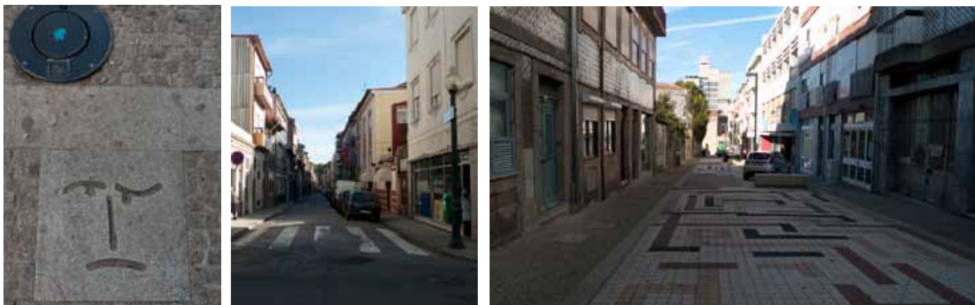
Fig. 1 and 2: The requalification of a segment in Miguel Bombarda Street, in 2009, included its pedestrianisation, new urban furniture and new pavement design by artist Ângelo de Sousa. Note (Fig.3) the fracture between the intervened area with the rest of the street. (Source: author's images, 2010)
