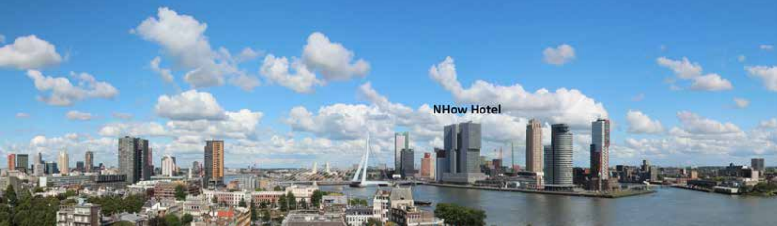
Figure 9. View of the Nhow Hotel in Rotterdam Source: Google Earth; and panorama of Rotterdam with its towering landmarks. Source: Bic (Wikimedia Commons)
