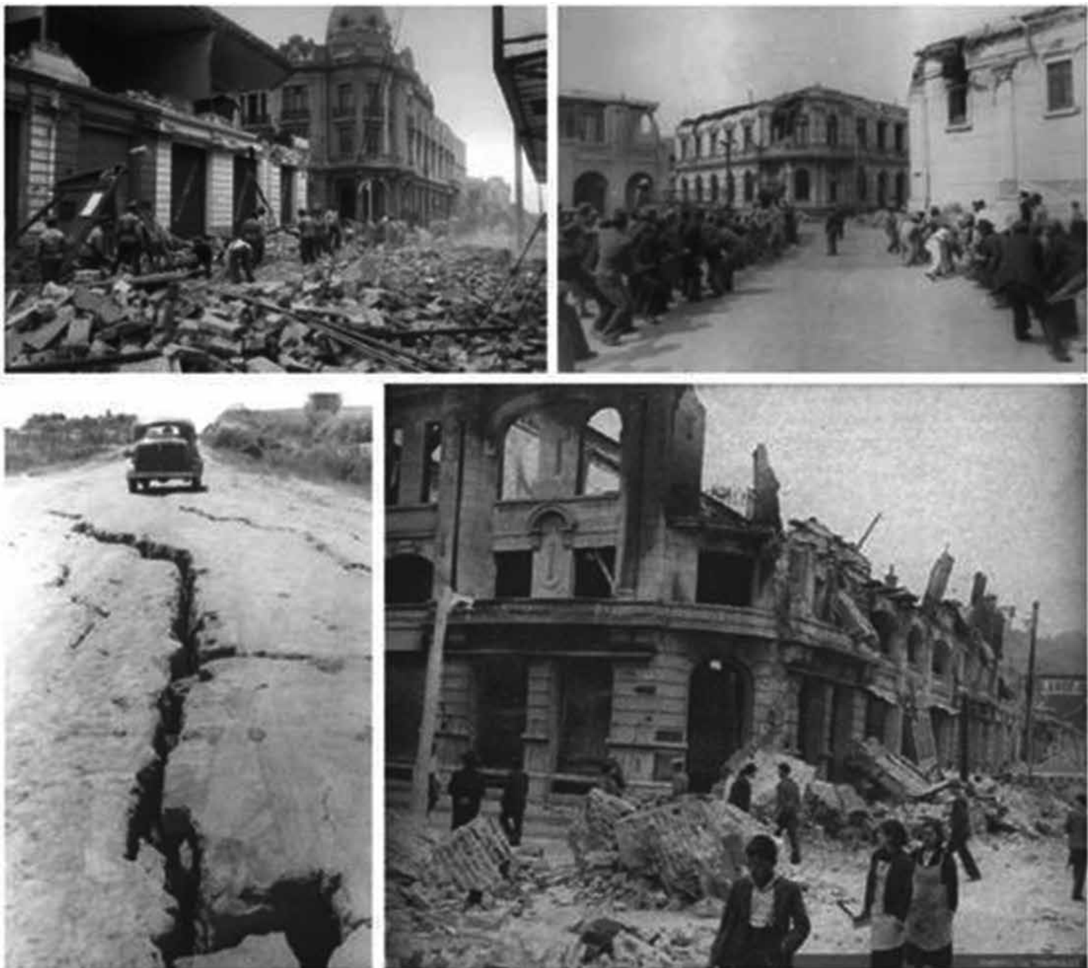
Figure 3. Earthquake in Concepción, 1939. Source: Photographic file, Sr. Alejandro Mihovilovic. Municipal library Concepción
